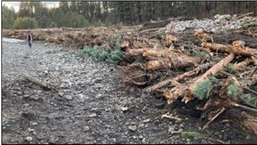
FIGURE 6 ROUGHENED EDGE BANK TREATMENT IN SIDE CHANNEL 5
